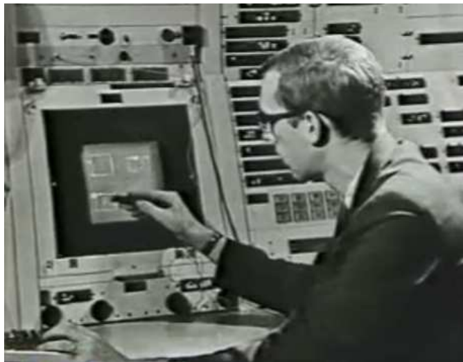
Figure 2-1: Sutherland's Sketchpad CAD application; still image from a demonstration video recorded at MIT Lincoln Labs in 1963.
