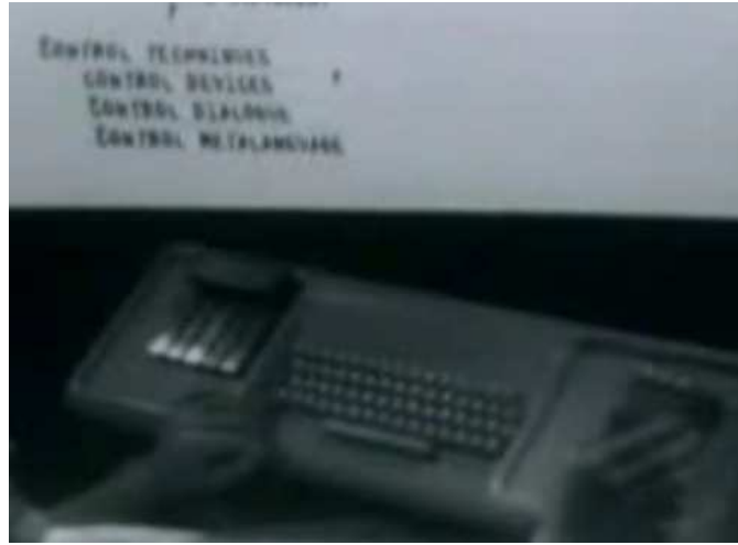
Figure 2-2: A still image from Doug Engelbart's demonstration video at SRI in 1968; this is the first time the mouse was shown to the public (in Engelbart's right hand).
